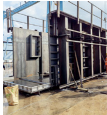
External formwork and framework 外模架
