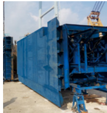
Internal formwork and framework 内模架
